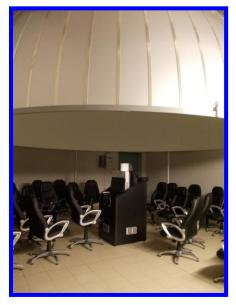
This dome is built to be installed at internal environments made exclusively to planetary use, consequently fixed construction. The manufacturing is done by semispherical sections, solution that allows the transportation and entry to destination to install directly in the final place.
