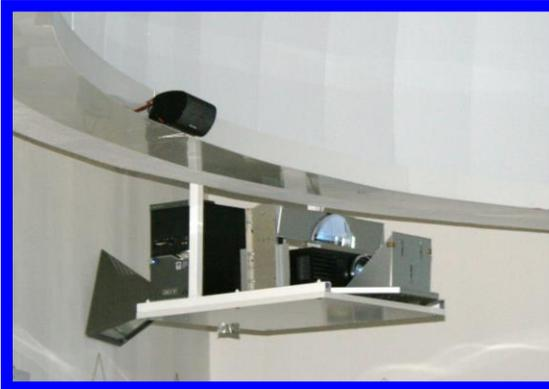
It's a digital projection system with images of composition of projectors. All dome is illuminated by the composition of 2 high resolution projectors that are part of the special system of video projection, composed set of special optics located centrally in a single block or at the sides of the dome divided in two parts leaving free the middle. The combination of this system through a "mosaic" compose
