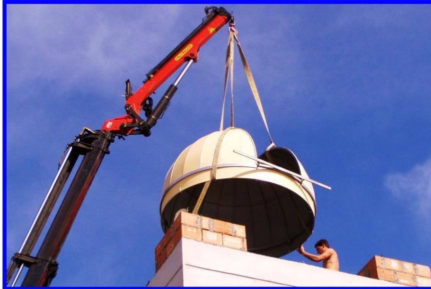
Example of dome installation, diameter 240cm over a roof.
