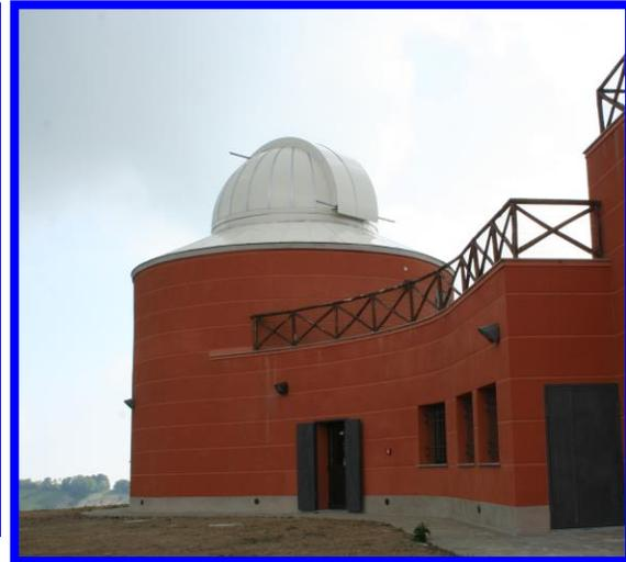
The construction of the structure in rotation and the base it's done in galvanized metal pipe then it's covered with aluminum sheets. The color of the dome can be chosen according to different proposals of the RAL which are offered to clients.
